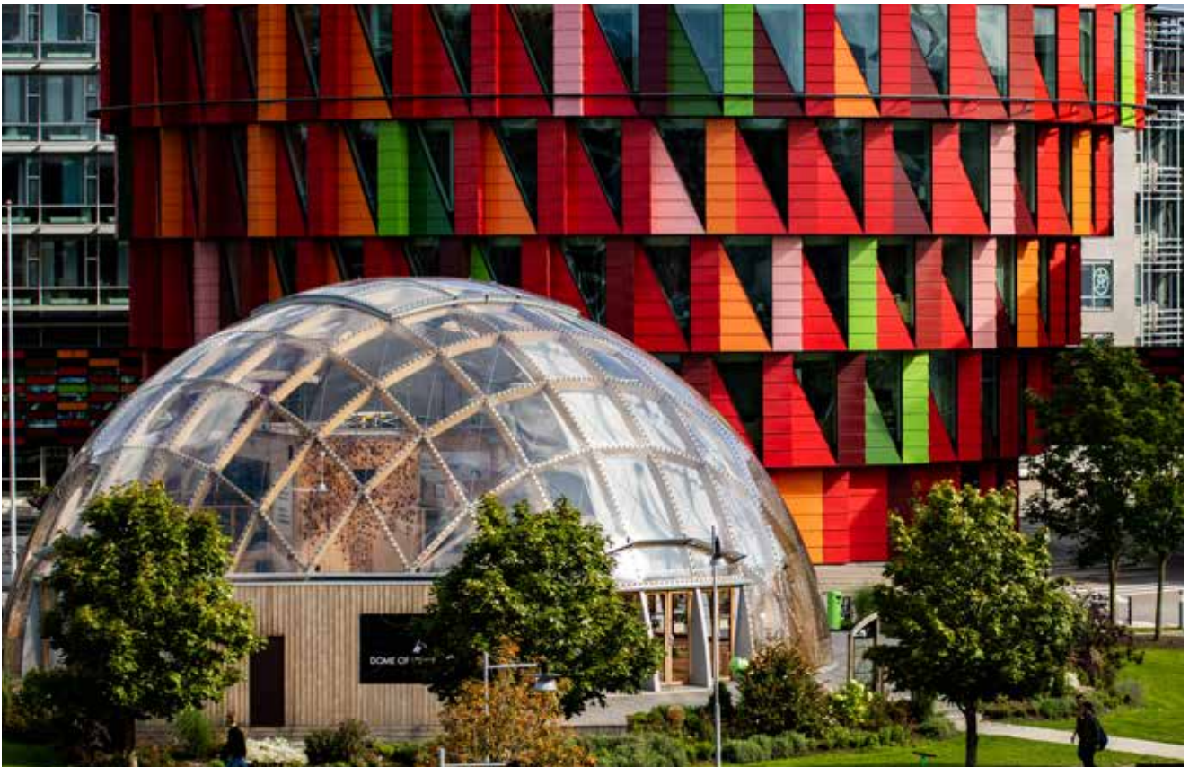
The "Dome of visions" was opened in 2018 at Lindholmen in Gothenburg. One function of the dome-shaped building is as a meeting point for conversations about sustainability.
